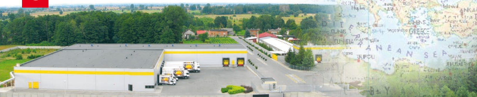
The Ovovita facilities are located in Prawda in the Lodz region.
